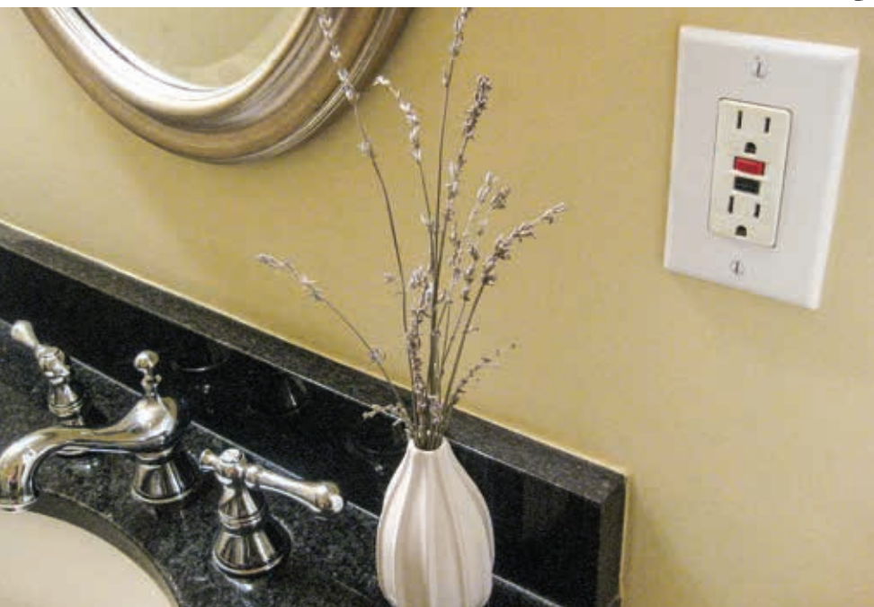
A GFCI should be used in any area where water may come into contact with electrical products, such as the bathroom, kitchen or outdoors.
