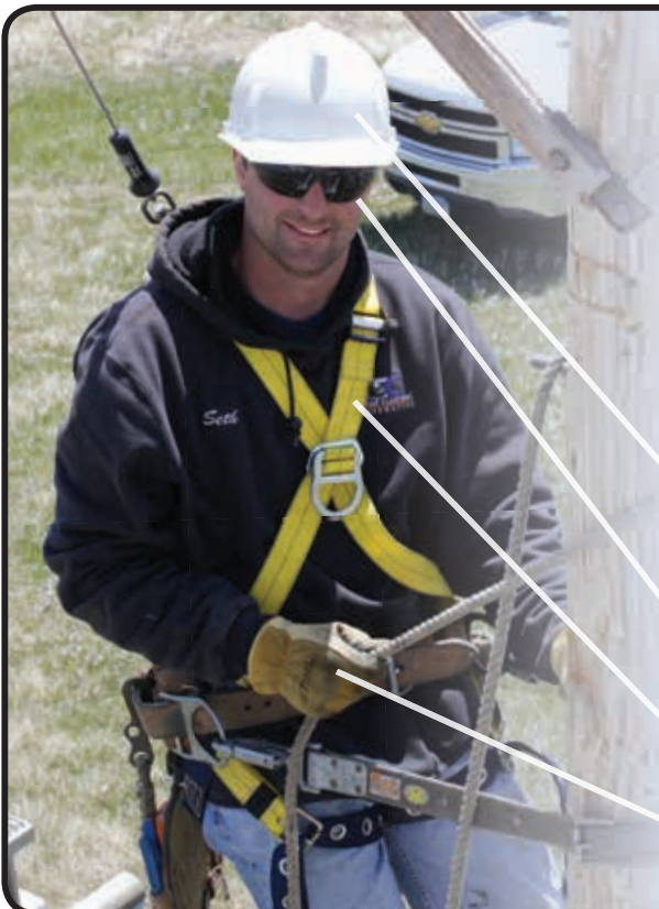
Brad Johnson , lineman for Capital Electric Cooperative, pounds a screwdriver into the pole. In the event he would be working on a single-phase distribution line that would not have a cross-arm, he could secure the rope with his screwdriver before lowering an injured person to the ground. Jason Smith , safety instructor for NDAREC, watches from the ground to make sure Johnson performs the rescue safely.
