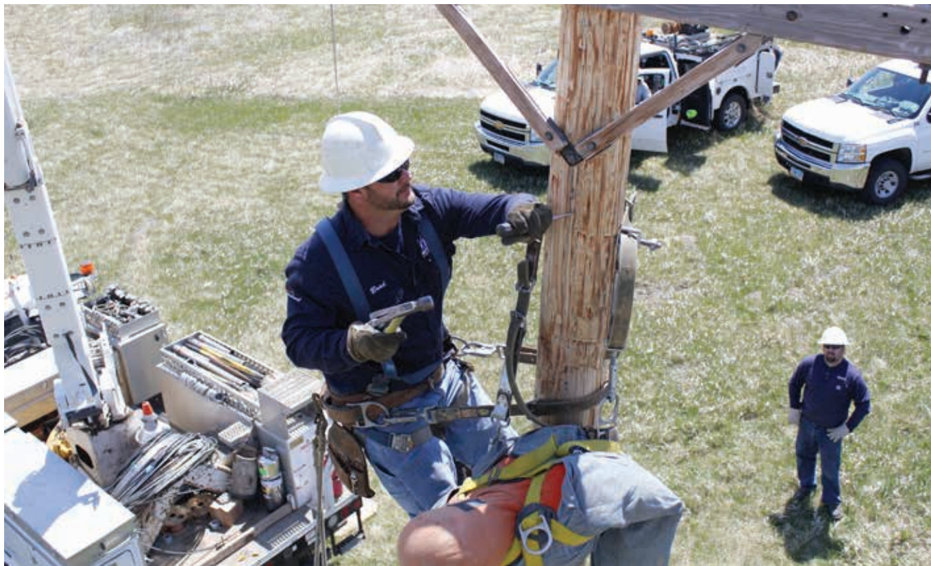
Brad Johnson , lineman for Capital Electric Cooperative, pounds a screwdriver into the pole. In the event he would be working on a single-phase distribution line that would not have a cross-arm, he could secure the rope with his screwdriver before lowering an injured person to the ground. Jason Smith , safety instructor for NDAREC, watches from the ground to make sure Johnson performs the rescue safely.
