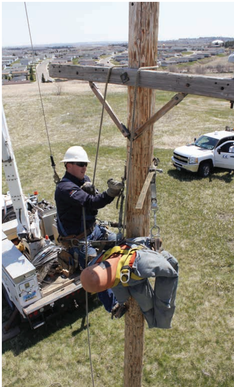
Jeff Holzer , lineman for Capital Electric Cooperative, uses the pole's cross-arm to secure the rope.
