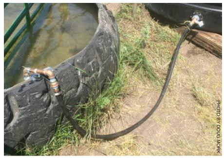
A simple gravity flow piping system is used to feed the drinking tank from the storage tank. A mechanical float valve closes when the drinking tank is full, allowing the solar pump to refill the storage tank. An electrical float valve in the storage tank shuts down the solar pump.
