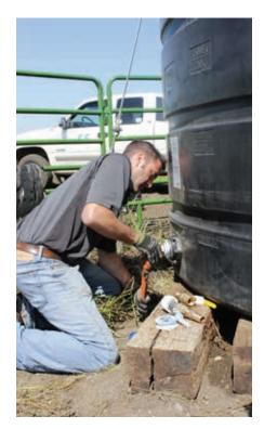
Josh Schaffner connects the gravity flow piping and valves for the drinking tank. The storage tank can hold 4,000 gallons of waters. If the cattle consume large amounts of water on extremely hot days, the pump may not keep up without using a storage tank. When a mechanical float valve in the drinking tank opens, water flows from the storage tank. The pump starts when the level in the storage tank drops and will continue until both tanks are full.
