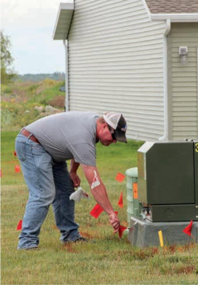
When converting from overhead to underground, the cooperative's staking department first plans the route in which to lay the cable. Here, Assistant Staking Engineer **Beau Townsend** shows how he places white flags in the ground to mark the route a contract crew will follow to trench or bore the powerline.
