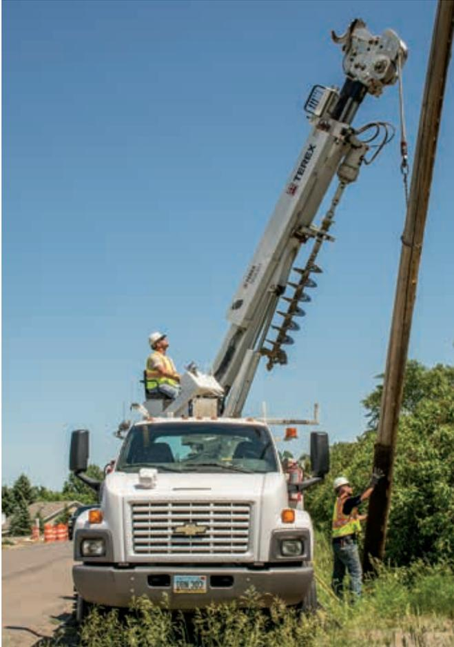
After the overhead conductor was removed, Journeyman Lineman **Steve Kuball** clamped the pole with a set of claws to control it. Journeyman Lineman **Matt Hagen** wrapped a cable from the winch around the pole, and the digger/derrick pulled the pole from the ground.
