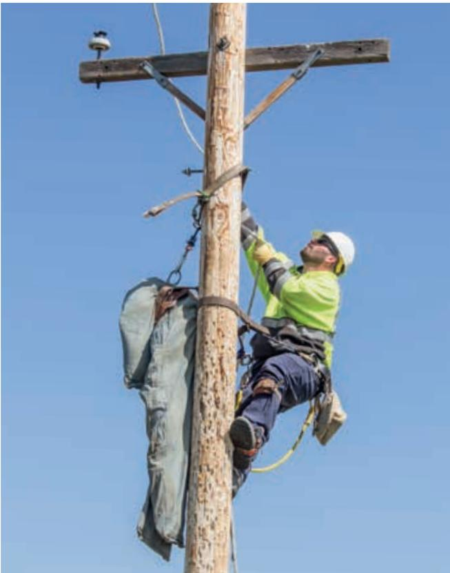
**Charles Atkinson**, lead lineman in Wing, throws his rope over the cross-arm in order to secure it, before threading it around the body of the mannequin.
