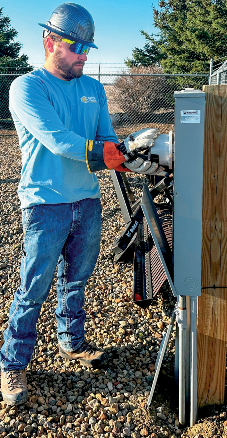
Journeyman lineworker Braden Martin replaces an existing two-way automatic communication system meter with a new digital wireless meter.
