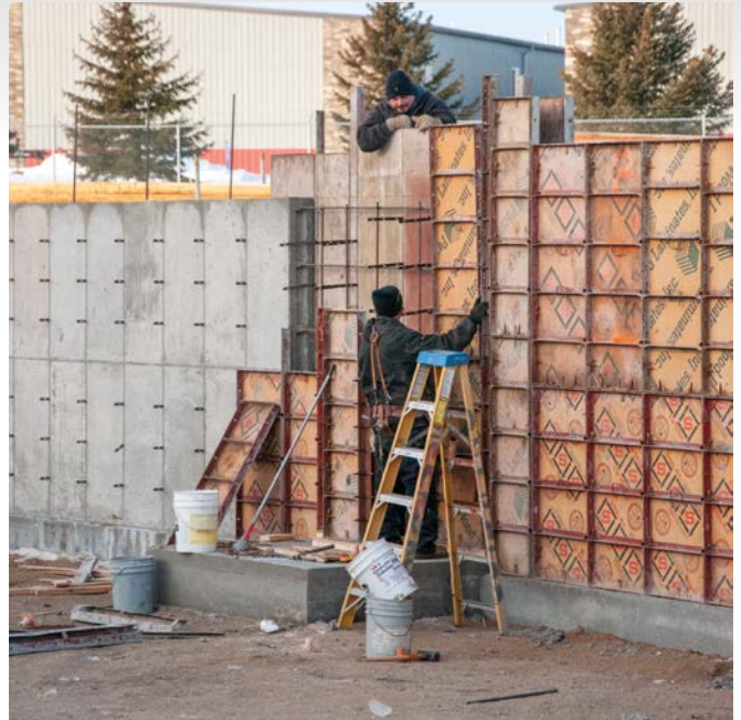
Construction is underway on a 10,000-square-foot storage building, which will be completed in 2023.
